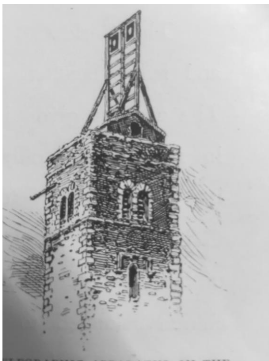
Clock Tower showing the semaphore mechanism installed during the Napoleonic Wars F. G. Kitton, SAHAAS
