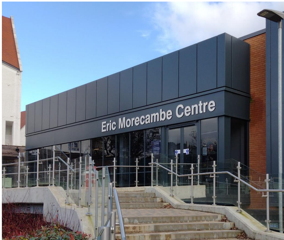
Eric Morecambe Centre, converted from previous Sports Hall and replacing the Public Halls. Opened October 2021.
